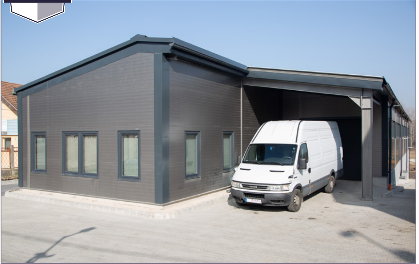
Restoration office and workshop hall 12 m x 45 m x 4,5 m | Place of fulfillment: Pécel
