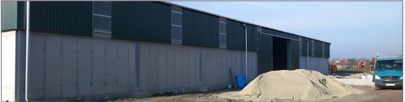
Agricultural warehouse 20 m x 48 m x 5 m | Place of fulfillment: Szigetcsép
