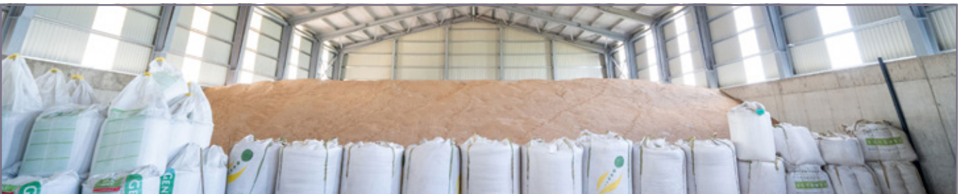
Crop storage hall with front roof | Place of fulfillment: Medgyesegyháza
