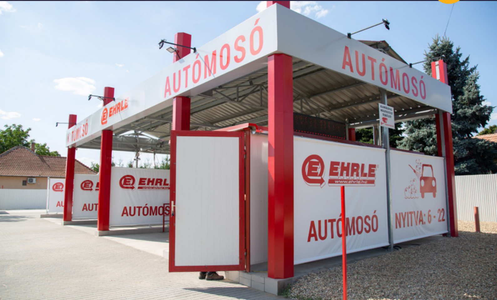
Light structure car wash building with 3 stations | Place of fulfillment: Heves
