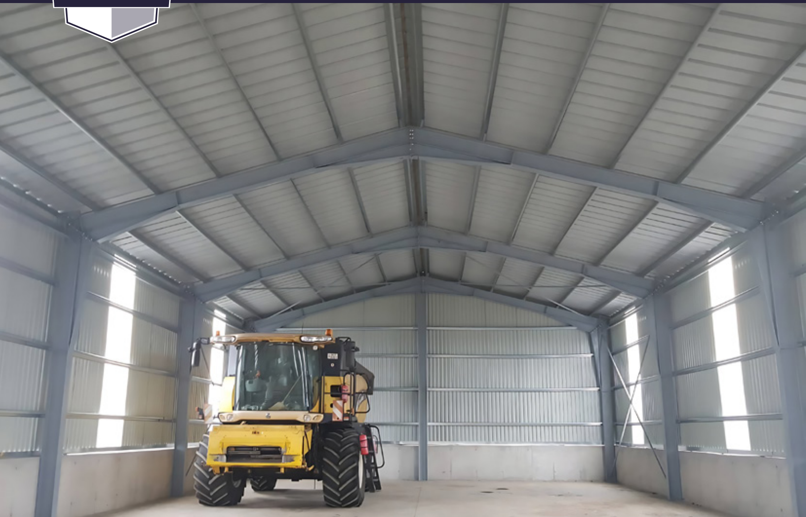
Machine and crop storage 13 m x 24 m x 5 m | Place of fulfillment: Detk
